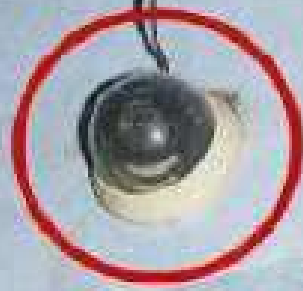
CCTV Camera No. 4
